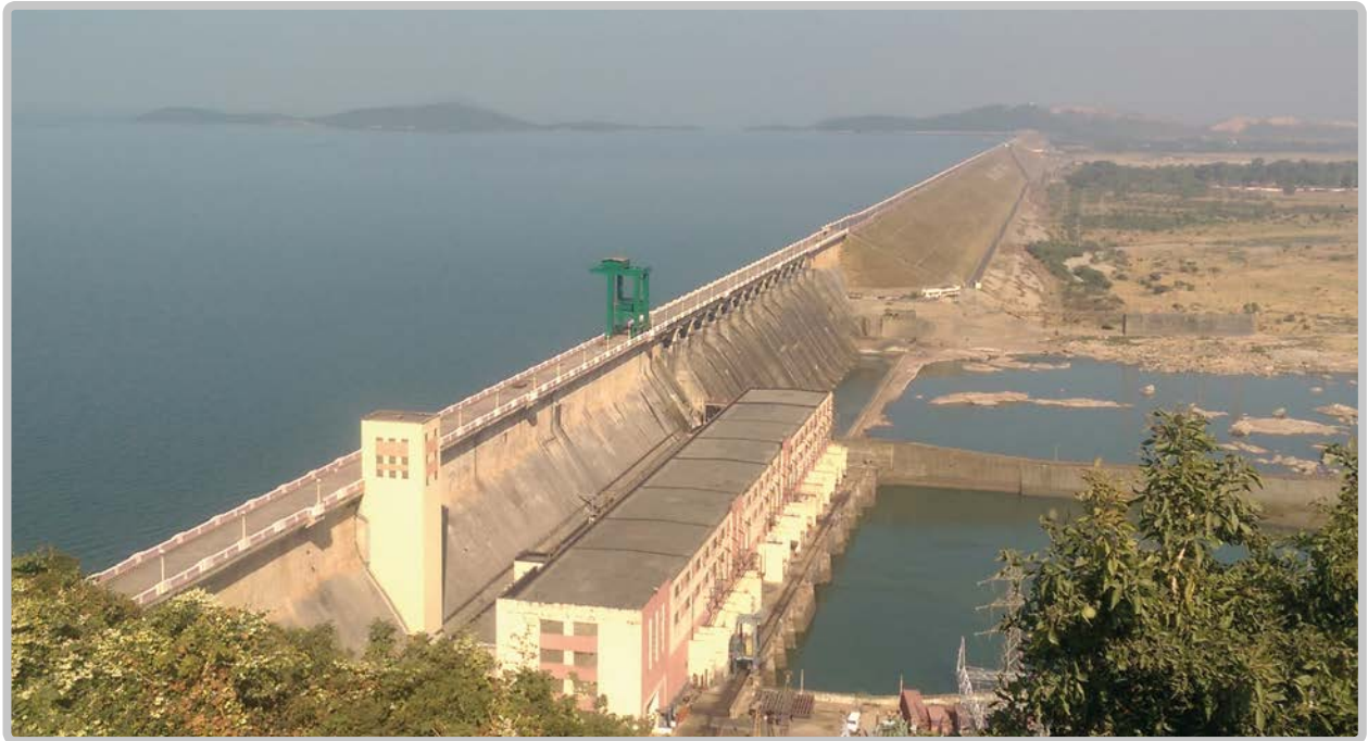
Hirakud dam on Mahanadi river, Odisha, India.
