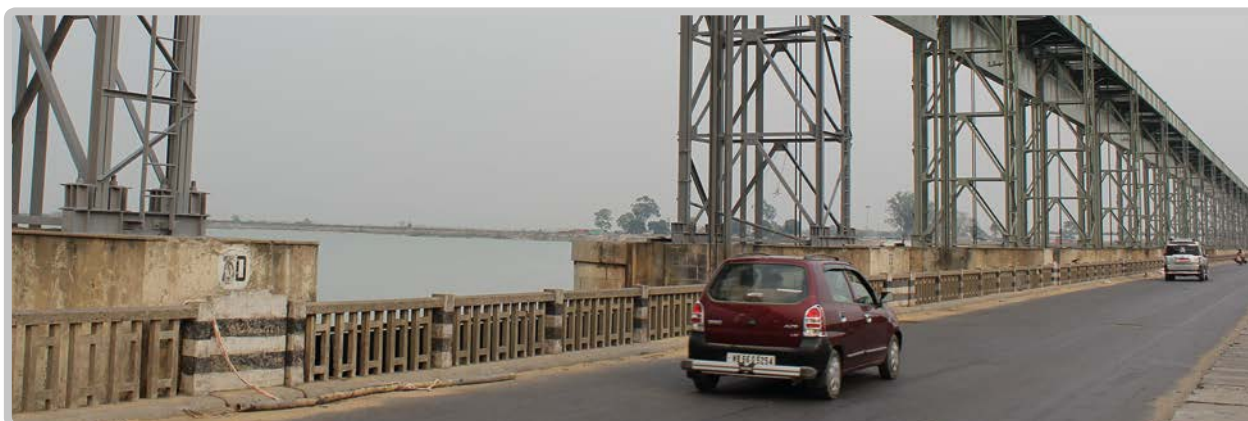
Water management structure over bridge in Patna, Bihar, India.
